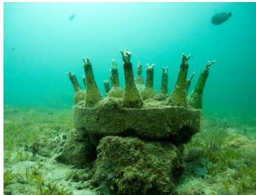
Figure 4. Bottle reef: a concrete structure holding 16 glass bottles that are used to hold corals.
